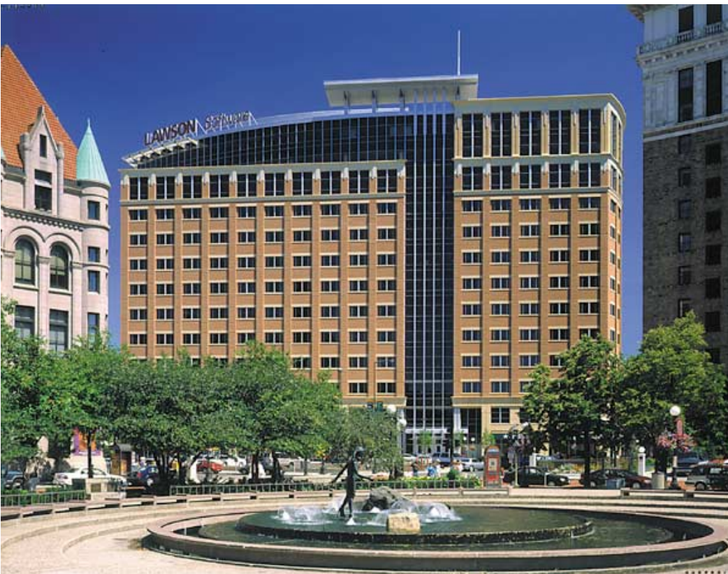
Lawson.Commons: a forward-looking business finds its place in an historic neighborhood
